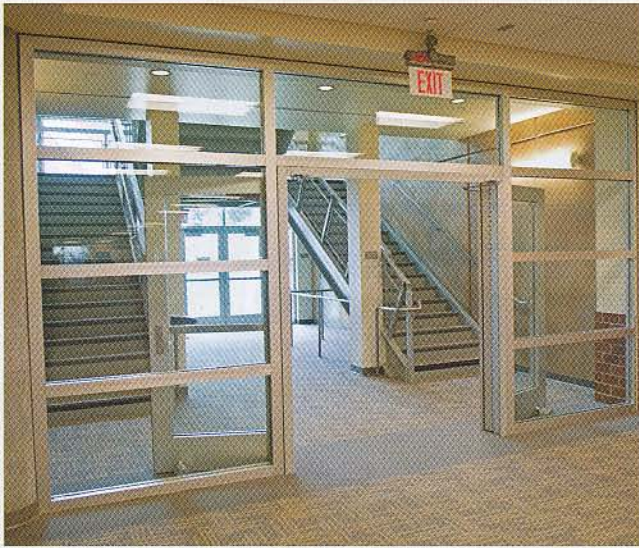
This 60-minute, temperature-rise door assembly at California State University, Fullerton, has glazing and a frame that are both tested to meet the ASTM E 119 standard.
