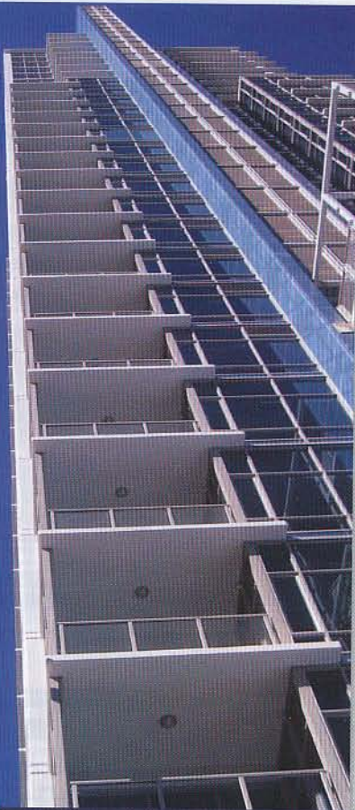
The property line of Sapphire Towers, on the right, forced architects and owners to use fire-rated glass to meet building codes.
