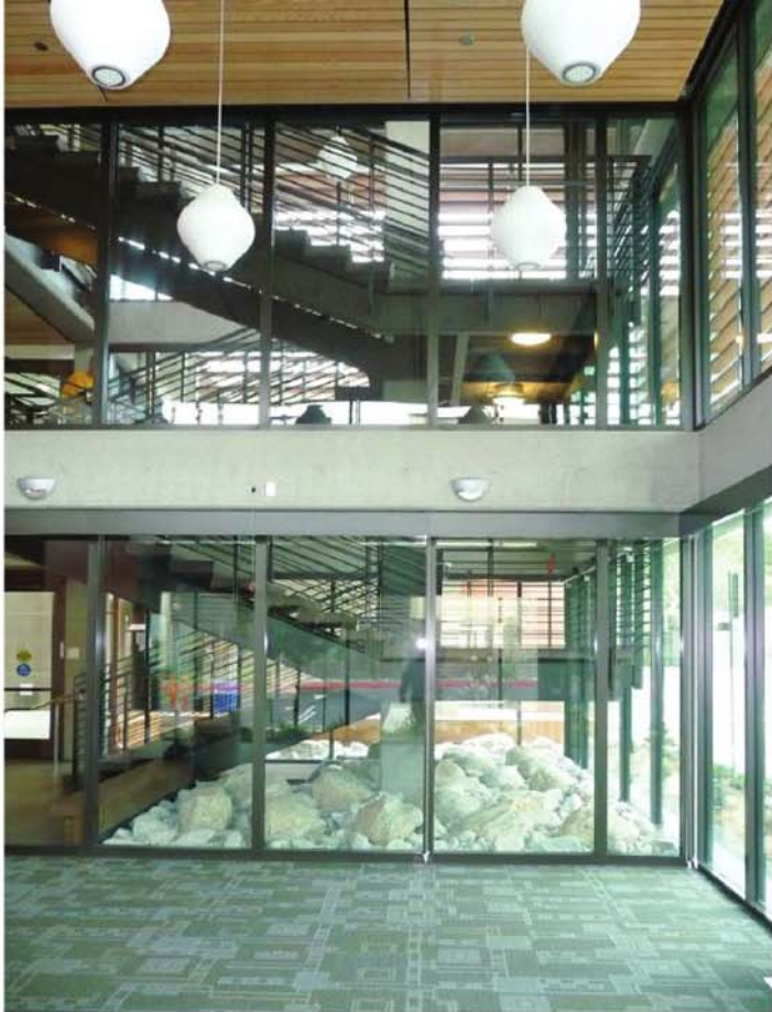
To enable natural light to penetrate further into Pomona College (California), clear, fire-rated walls were supplied. The system meets ASTM E 119/UL 263/NFPA 251 requirements for a two-hour stairwell enclosure.
