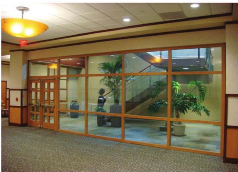
This two-hour fire-resistive protection stairwell at the Reid Hospital (Richmond, Indiana) meets ASTM E 119/UL 263/NFPA 251, Standard Test Method for Fire Tests of Building Construction and Materials .
