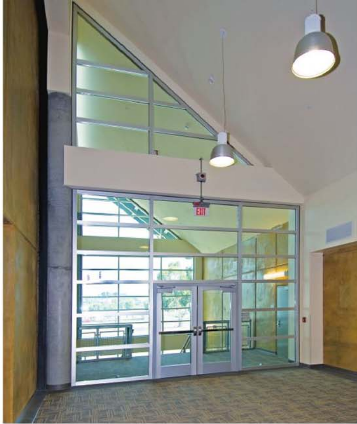
The framing system at CSU Fullerton Recreation Center (California), matched the non-rated systems used in the building's exterior, providing the uniform, seamless look the architect desired.
