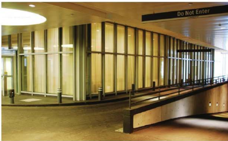
At Weill Cornell Medical College in New York City, the architect wanted an exterior curtain wall system with large glass lites wrapping around the building. However, this area leads into a parking garage, which needed to be fire-rated. To achieve the desired transparency, and meet the building code requirements, a two-hour fire-resistive curtain wall was installed.
